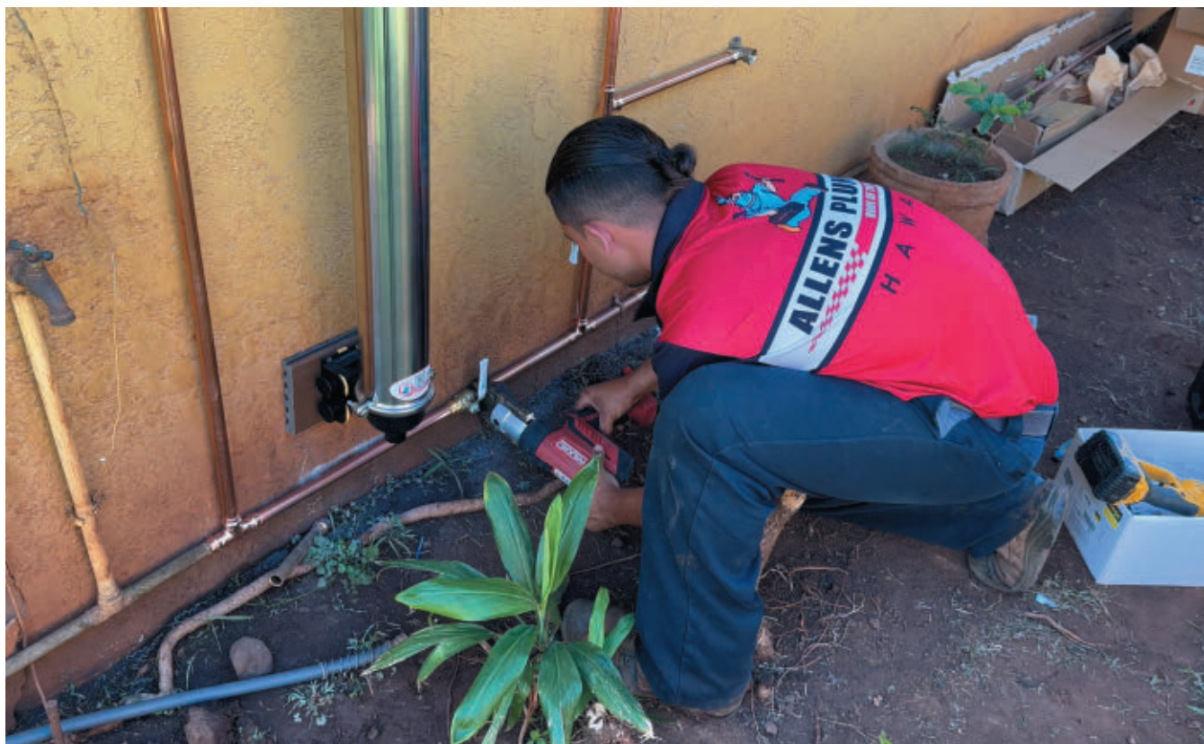
Allens Plumbing employee Sam installs a water filter in Lahaina.
